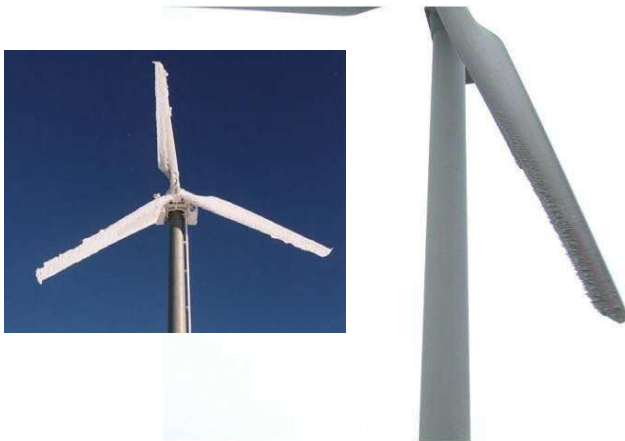
Ice formation on windmill rotor blades
